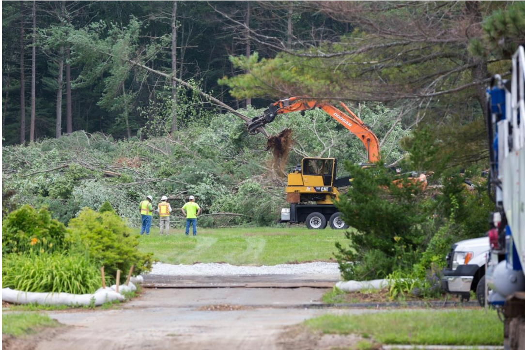
Tree Clearing Begins, July 12, 2017
