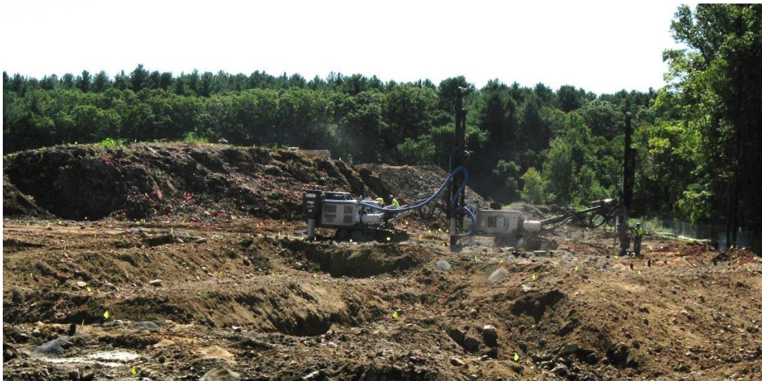
Blasting Operations, September 8, 2017
